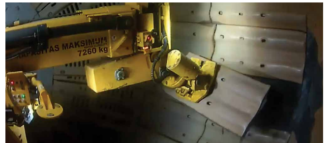
AFTER: Worn liners removed from the mill wall without crew inside
