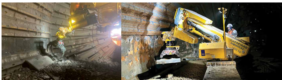
The RUSSELL Claw eliminates risks for reline crew members working on the charge inside the mill, enabling safer and faster removal of worn liners.
